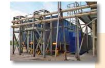
Bulk filling trailers are one of the options available for chip collection. Comprising of reverse onto fill pipework the system has auto fill sensors, trailer changeover diverters, docking steelwork.
